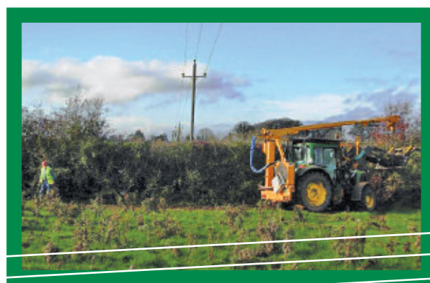
Figure 7.1 Hedge cutting beneath overhead electricity lines
